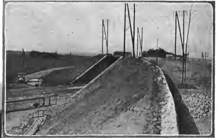
Spot on the main road from Paris to Fontainebleau at which a dangerous grade crossing existed. This has now been abolished by the P. L. M. Railroad Company building a bridge over the line
